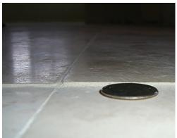
tion contractor can grind the tile to flatten the floor.
