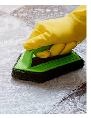
One of the biggest problems with epoxy grouts is failing to clean up the grout residue. Unlike cement-based grouts that can sit for 24 hours, epoxy grout needs to be thoroughly cleaned within one hour or cleanup may prove difficult to impossible, depending on the surface type. If epoxy residue remains, the following procedure is recommended:
