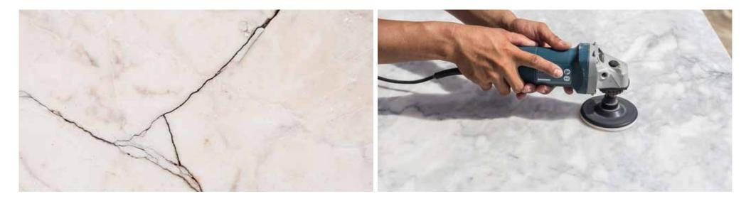
Crack and Chip Repair–Cracks and chips in stone can be filled.
