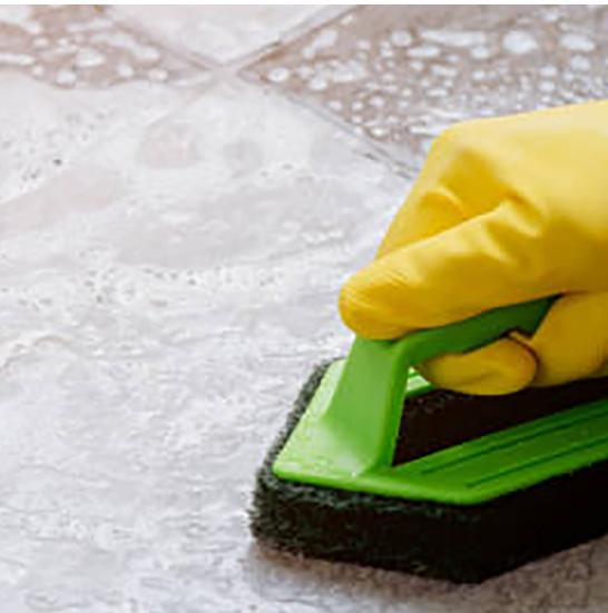
One of the biggest problems with epoxy grouts is failing to clean up the grout residue. Unlike cement-based grouts that can sit for 24 hours, epoxy grout needs to be thoroughly cleaned within one hour or cleanup may prove difficult to impossible, depending on the surface type. If epoxy residue remains, the following procedure is recommended:
