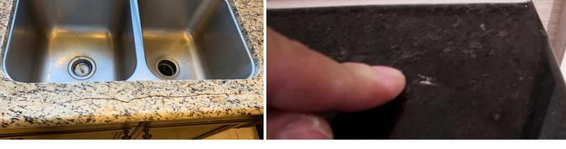
**Reparing Breaks**– Repairing breaks involves reattaching cracked or broken pieces of stone with specialized adhesives, filling any gaps, and blending or polishing the area so the repair is as seamless and structurally secure as possible.
