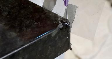
der by a craftsman who is experienced in their use. This is followed by a careful polishing technique that can only be mastered through experience. A restoration professional will also take care to protect the surrounding surfaces from damage. The diamond grinding technique involves using water and this could be damaging to wood and carpet if measures are not properly taken to protect these surfaces, walls, baseboards, appliances, etc.
